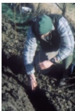
7. Placing plants along the edge of the trench prior to backfilling.
